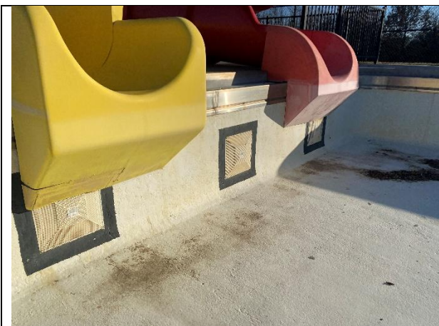
Figure 49 Waterslide suction inlets
