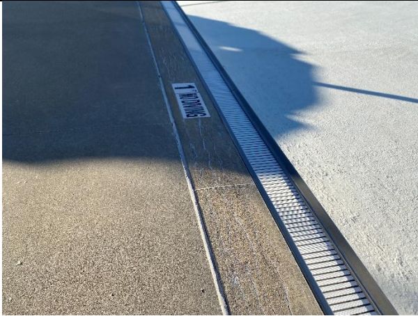
Figure 25 Pool gutter edge and deck
