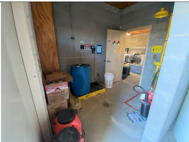
Figure 53 Acid storage room
