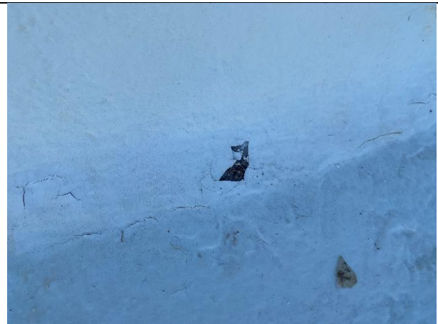
Figure 24 Exposed concrete wall at base of pool wall
