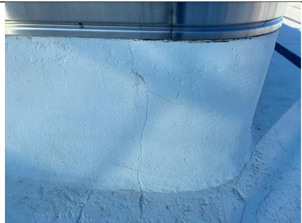
Figure 18 Vertical cracking on shallow end pool wall
