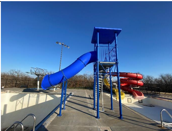
Figure 35 Sinking pool deck beneath deep slide
