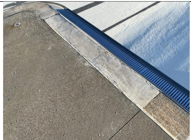
Figure 30 Area of deck to pool concrete transition
