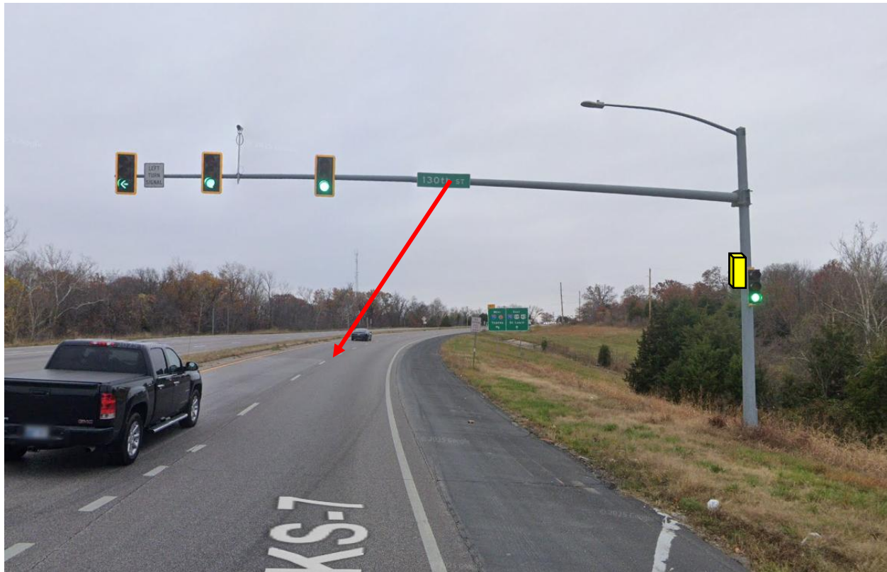
Figure 1: Facing North on KS-7 (October 2025) – Showing only the Northbound cameras.
