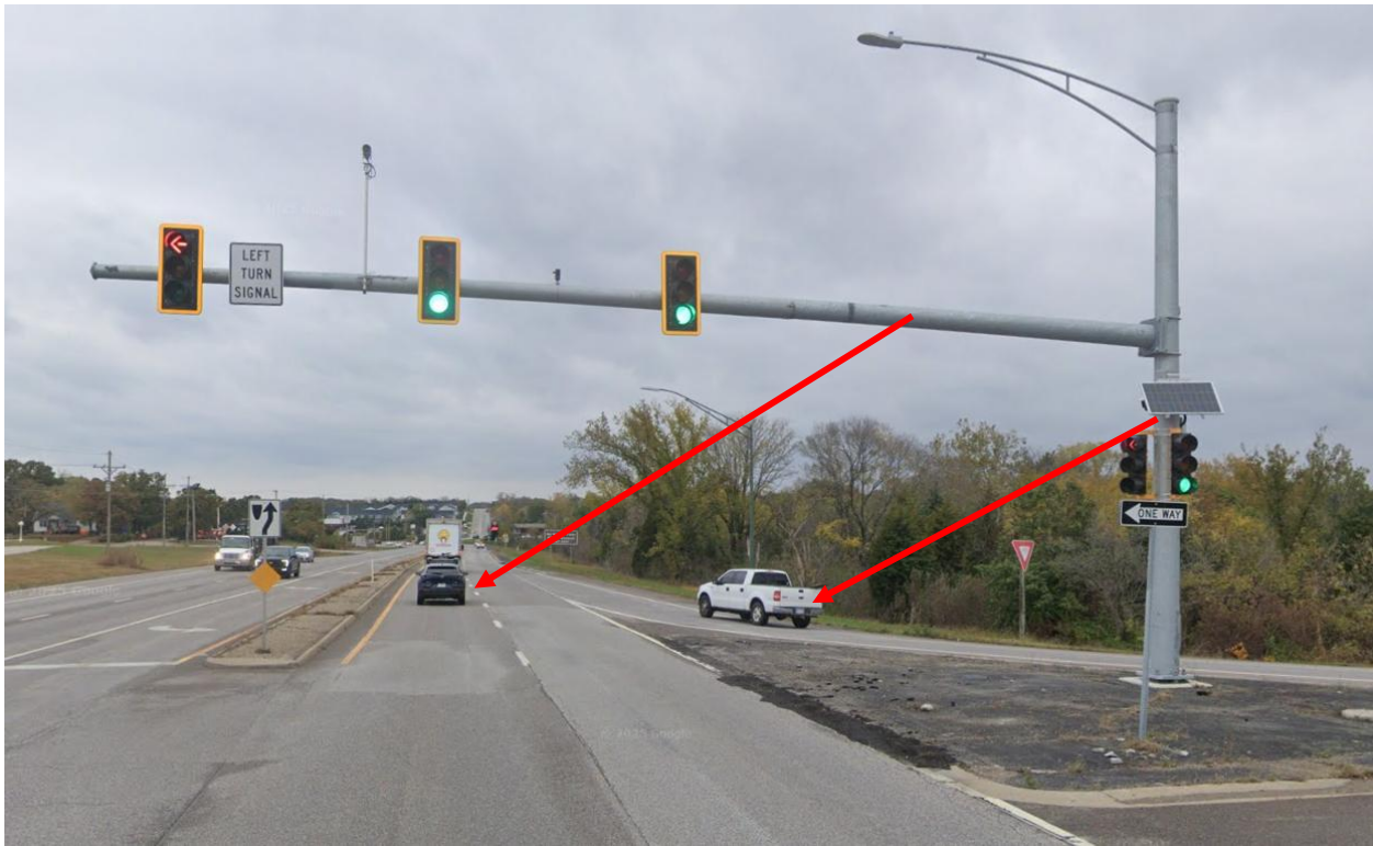
Figure 1: Facing North on KS-7 (October 2025) – Showing only the Northbound cameras.
