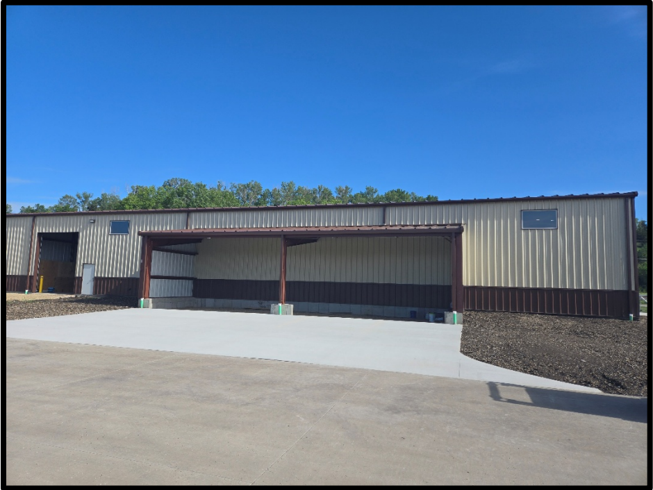
Concrete Overhang Area
