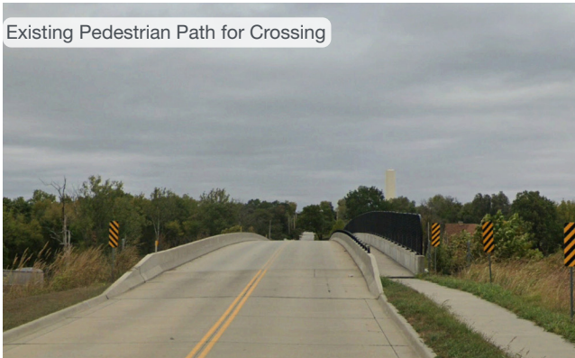
Crossing I - 70 at 118th Street
