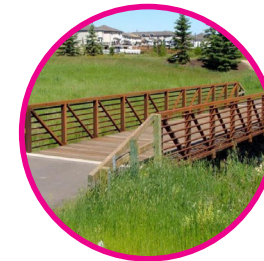
Small Pedestrian Bridge
