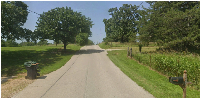
No Sidewalk on 122st St
