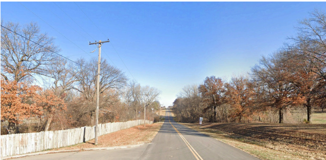
No Sidewalk on 126th St
