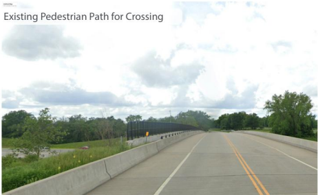
Crossing I - 70 at Riverview Avenue
