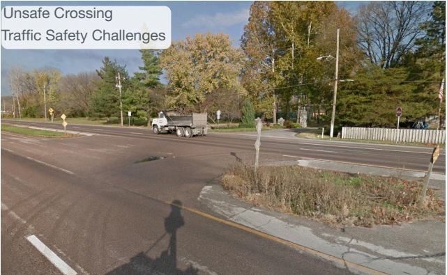
Intersection at K-32 and Lake of the Forest
