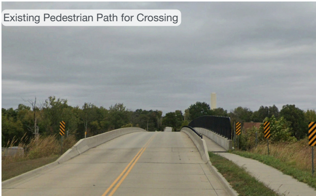
Crossing I - 70 at 118th Street
