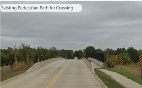
Crossing I - 70 at 118th Street
