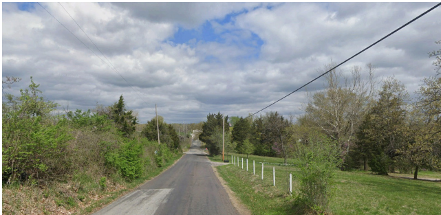
No Sidewalk on 118th St
