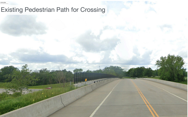
Crossing I - 70 at Riverview Avenue
