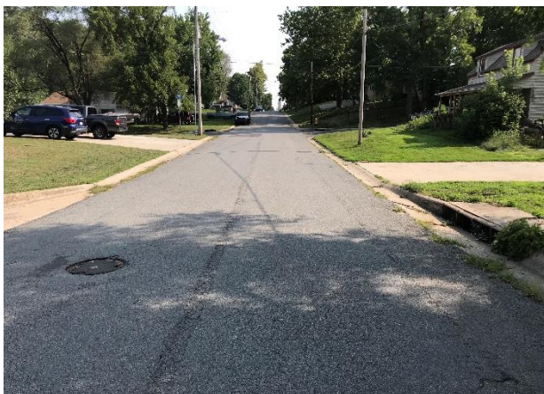
307 Emerson at Emerson curb inlet (Looking south)
