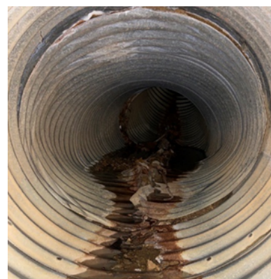
Junction of 60" CMP and 30" CMP
