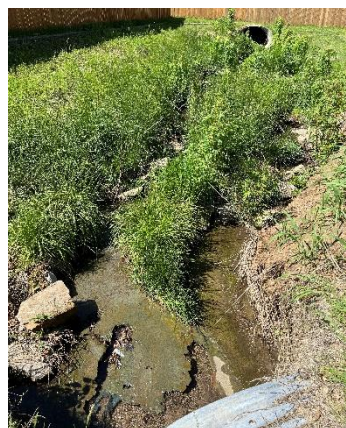
Open channel behind 307 Emerson at outlet (Looking south)
