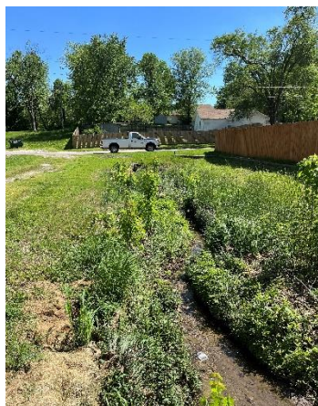
Open channel behind 307 Emerson at inlet (Looking south)
