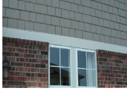
The brick sill is interrupted by a window.
