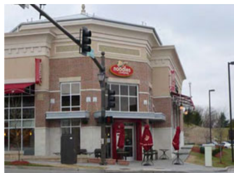
The stucco wall is located above the brick and stone wall; the brick and stone comprise at least 50% of the wall area.
