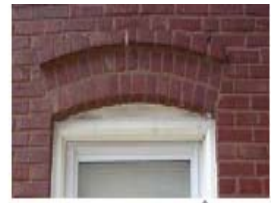
A segmented arch above a window opening.
