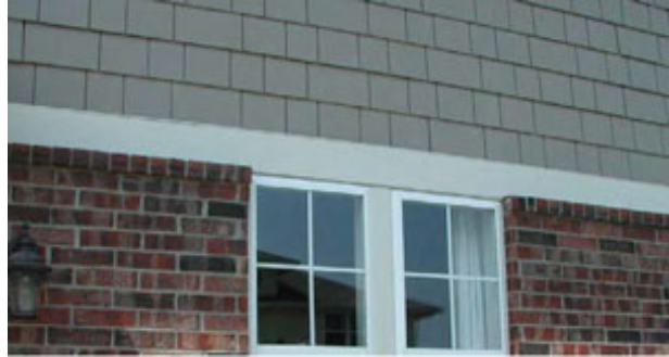
The brick sill is interrupted by a window.
