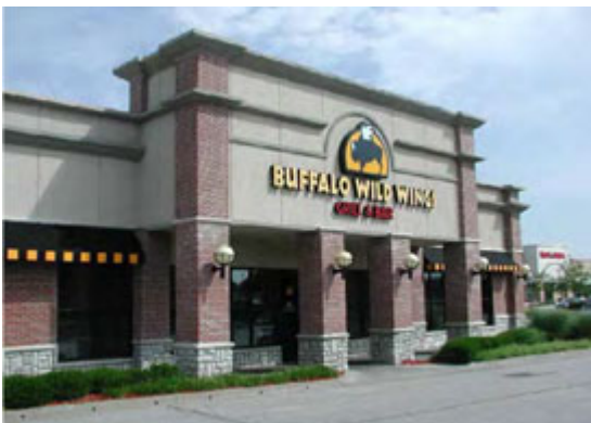
The customer entrance correctly contains columns, display windows, raised parapet, and recesses.
