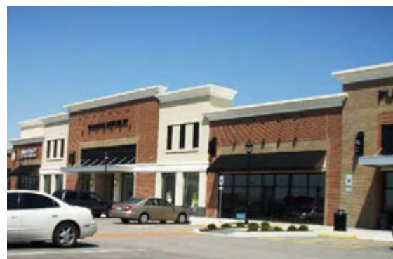
The parapet on this building modulates; cornices correctly return at least 8 feet at exterior corners.
