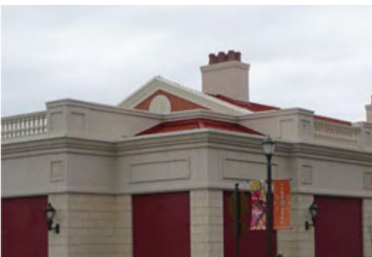
The parapet and cornice returns back into a pitched roof.
