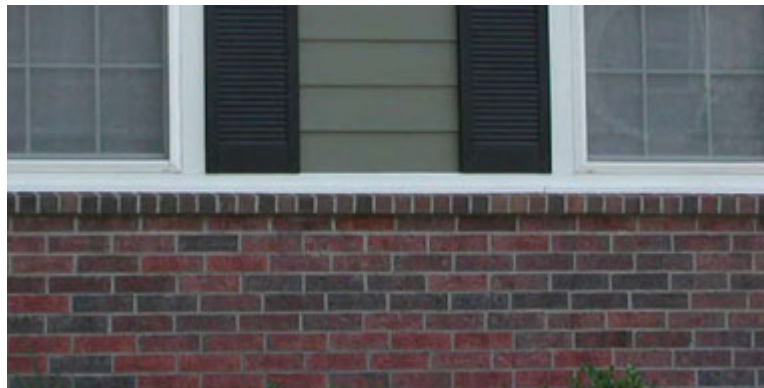
The brick sill is uninterrupted by wall openings.
