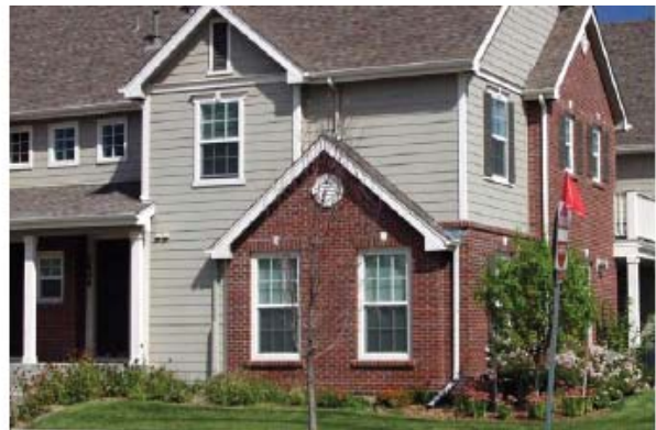
This vertical change in material is done correctly; it turns the corner and does not terminate within 4 feet of the corner.
