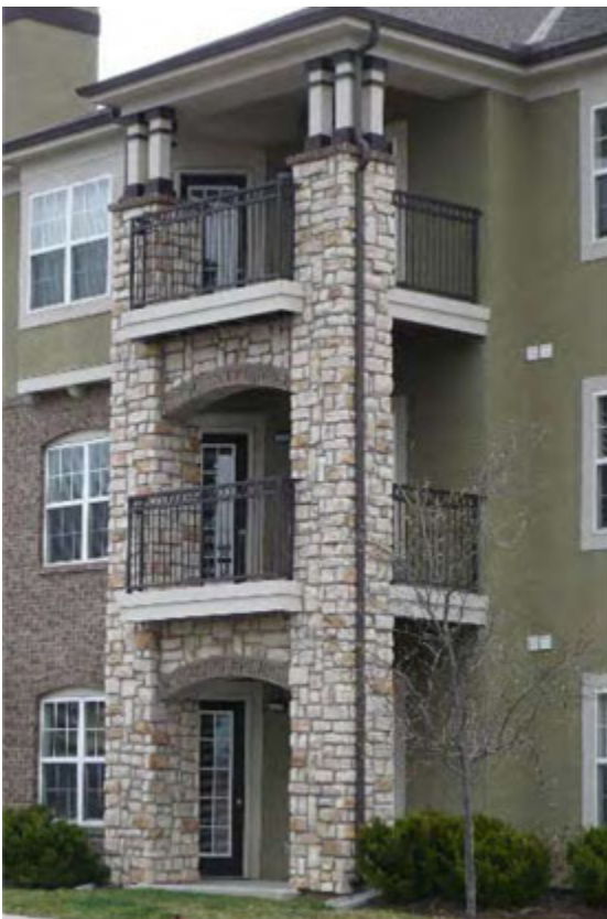
Porch with arches, iron railings, and columns.
