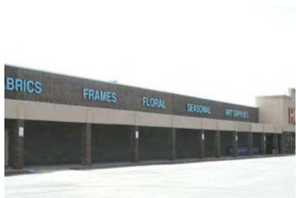
This building is over 50,000 s.f. and does not contain both pitched roofs and flat roofs with parapets.
