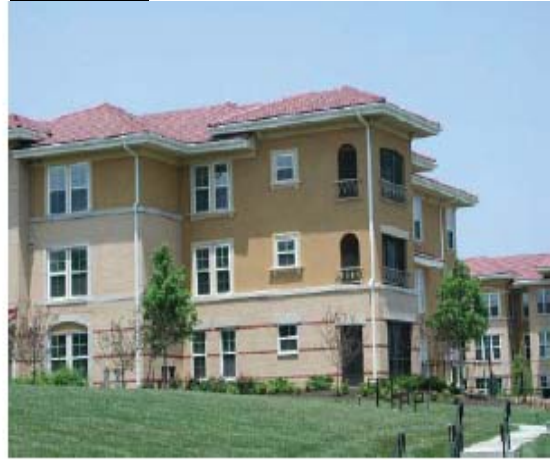
This taller apartment building still has the details of a single-family house.
