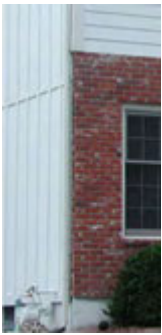
A vertical change in material occurs within 4 feet of an exterior corner.
