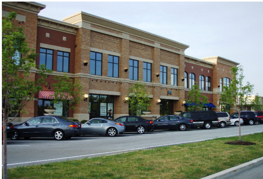
The building color consists of low-reflecting and subtle colors that complement the building details and materials.
