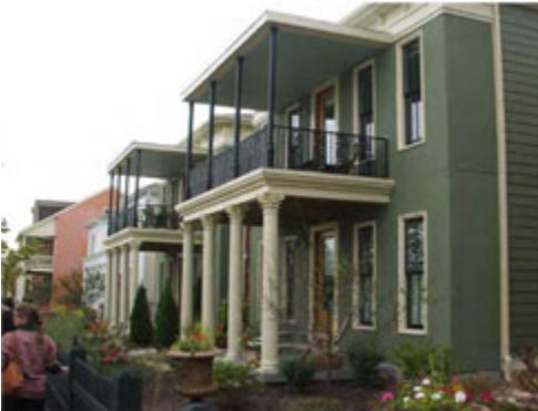
Front porch with balcony
