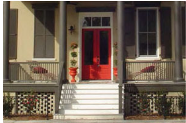
This front door is detailed with an transom and columns supporting a roof.
