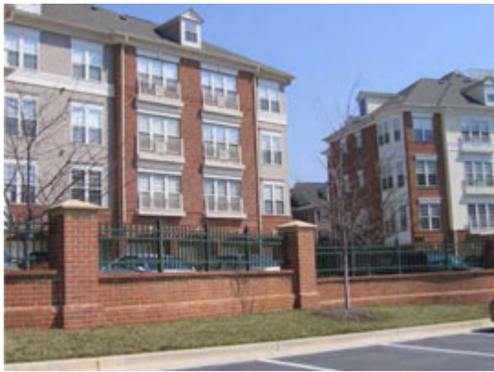
The vertical change in material correctly occurs at an interior corner; the siding is correctly located above the brick.
