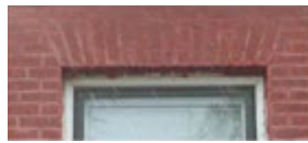
A jack arch above a window opening.
