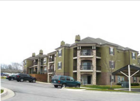
This building has consistent detailing on all sides.
