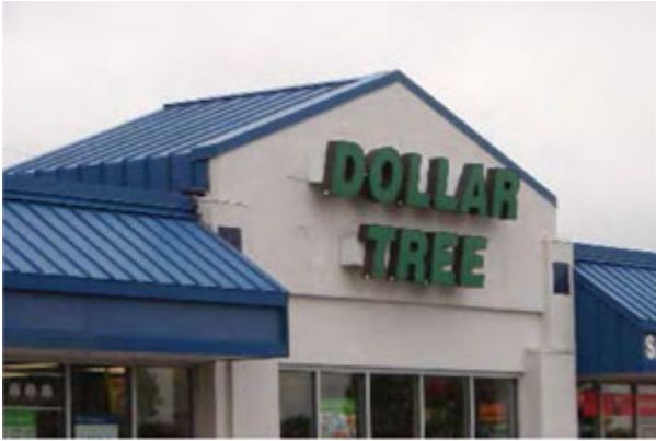
The pitched roof lacks any overhanging eaves.
