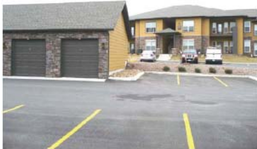
The garage's details and materials are compatible and consistent with the primary structure.
