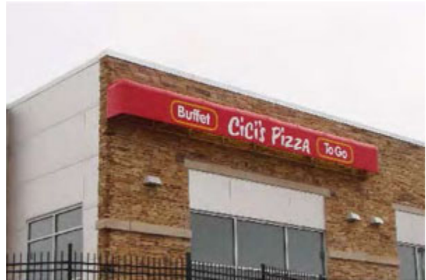
The awning is higher than the top of the window.
