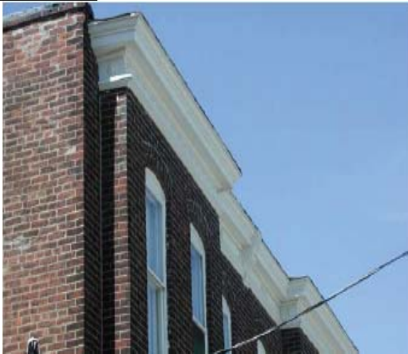
The cornice wraps around the entire building projection.
