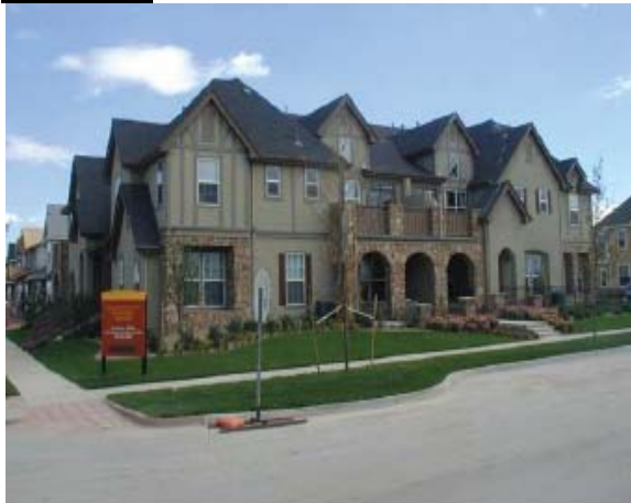
The arches, terraces, material, and trim of this apartment building gives it the appearance of a single-family house.
