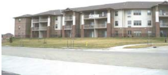
This apartment building is too long; its length is over 200 feet.
