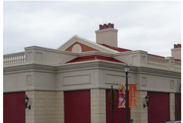
The cornice correctly continues around the entire building projection.
