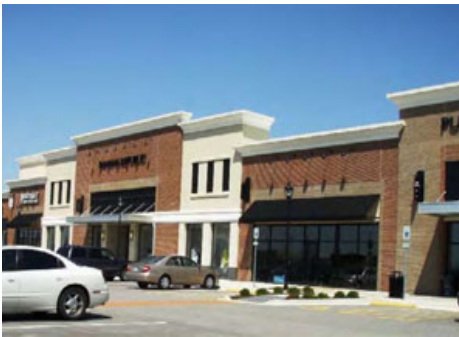
The brick comprises at least 50% of the wall area; horizontal changes of materials do not occur within 4' of an exterior corner.
