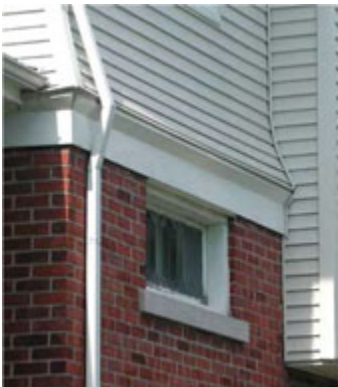
A horizontal change of materials with flared siding and trim.
