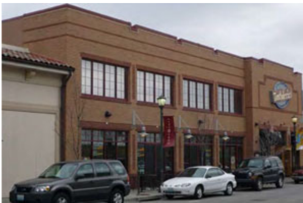
The second story windows align with the vertical bays from the first floor.
