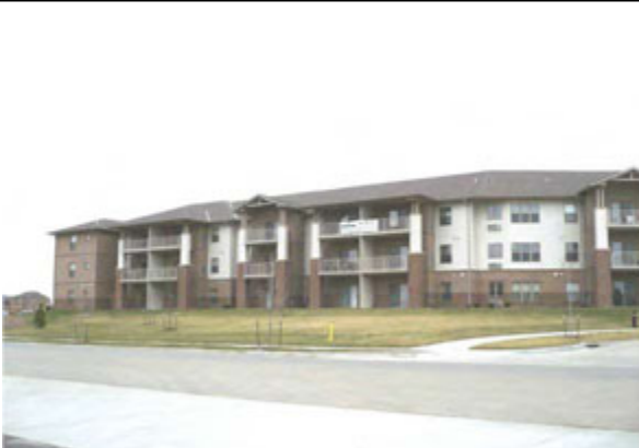
This apartment building is too long; its length is over 200 feet.
