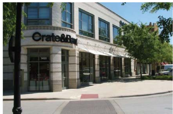
This customer entrance has adequate details; it contains awnings, display windows, overhangs, and recesses.
