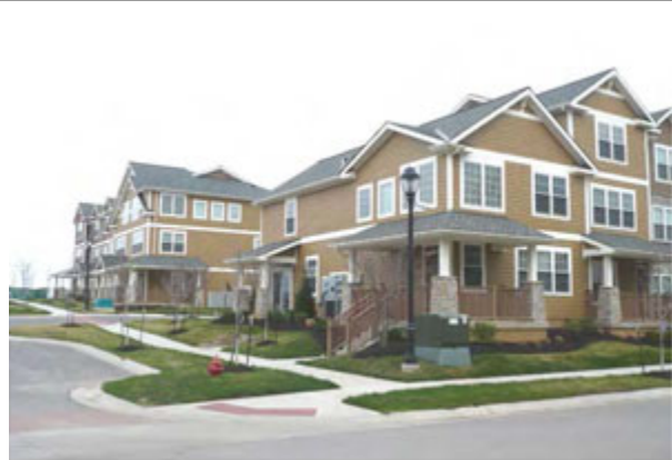
This building has the same detailing on all building walls.
