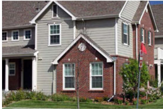
This vertical change in material is done correctly; it turns the corner and does not terminate with 4 feet of the corner.
