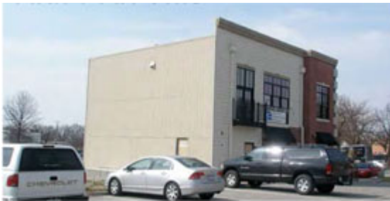
This building has no detailing on one wall.
