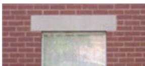
A stone lintel above a window opening.
