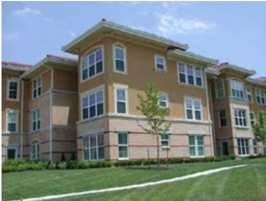
This apartment building correctly has stucco located above the stone.
