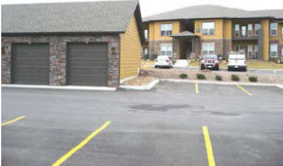
The garage's detail and materials are compatible and consistent with the primary structure.
