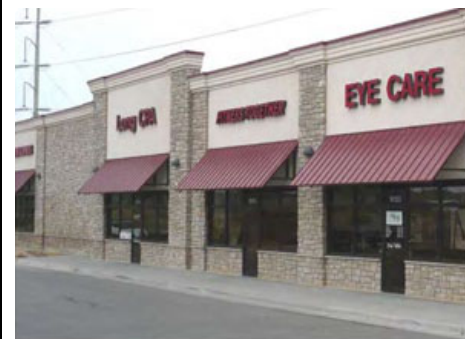
The stucco wall is located above the stone wall; the stone comprises at least 50% of the wall area.
