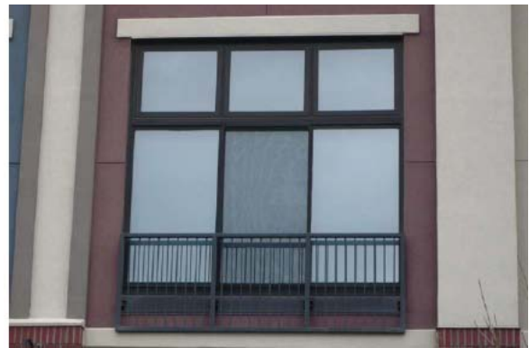
The window opening has a lintel and a sill.
