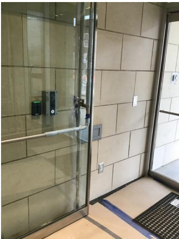
20201211_092943_photo Henderson Engineers Dec 11, 2020 9:29 AM
