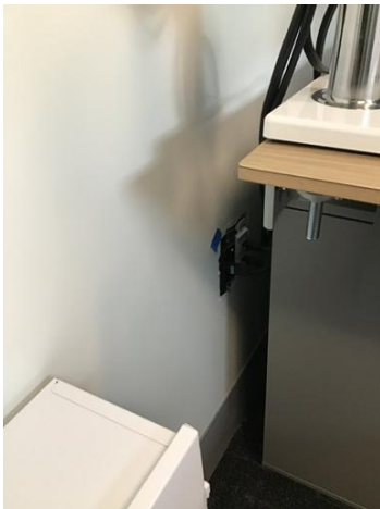
20201211_094114_photo Henderson Engineers Dec 11, 2020 9:41 AM
