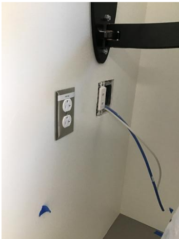
20201211_093729_photo Henderson Engineers Dec 11, 2020 9:37 AM
