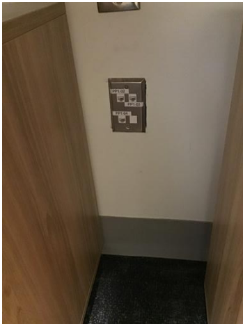
20201211_093615_photo Henderson Engineers Dec 11, 2020 9:36 AM
