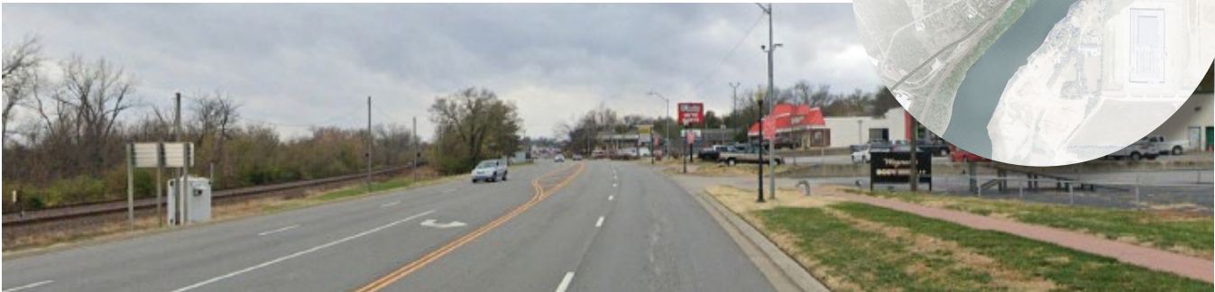
Existing Street B1
