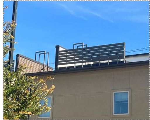
Figure 4.11. Roof-Mounted Equipment Screen
