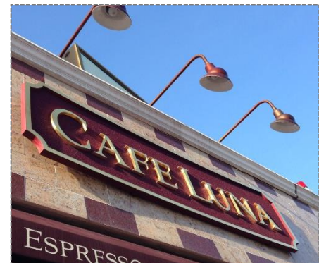
Figure 4.17. External Down Lighting
