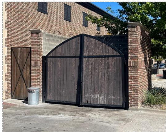
Masonry Screening Walls with Wooden Gate
