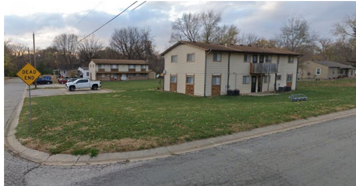
Figure 10. Highview Avenue and Park Street looking northwest at homes and apartments in the floodplain.
