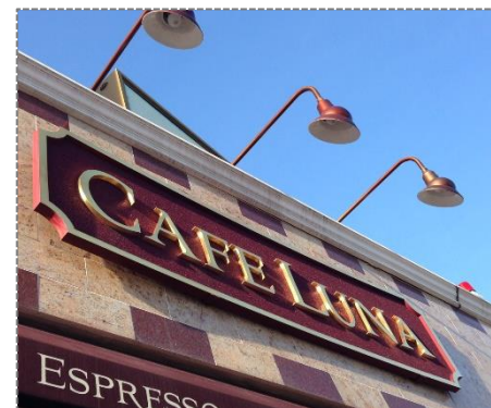
Figure 4.17. External Down Lighting
