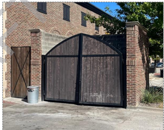
Masonry Screening Walls with Wooden Gate
