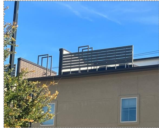
Figure 4.11. Roof-Mounted Equipment Screen
