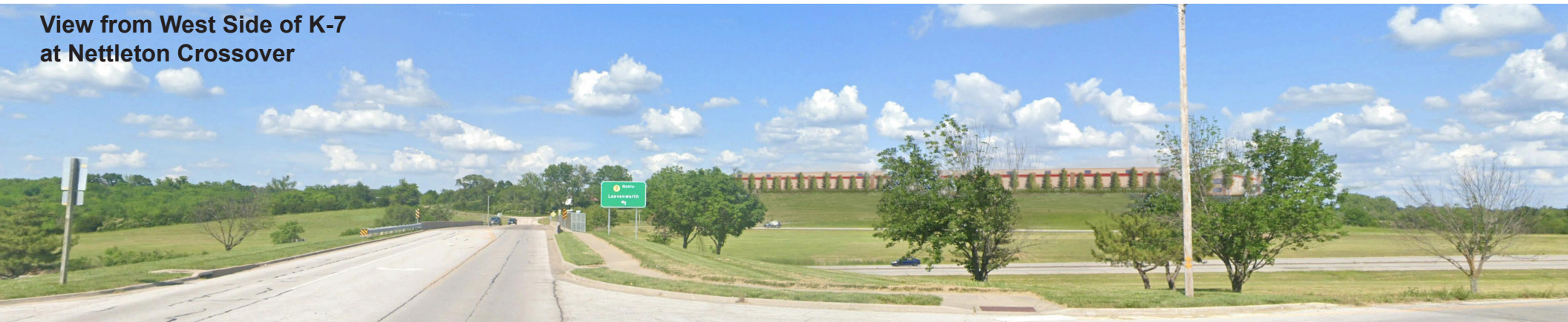
View from South K-7 Exit Ramp
