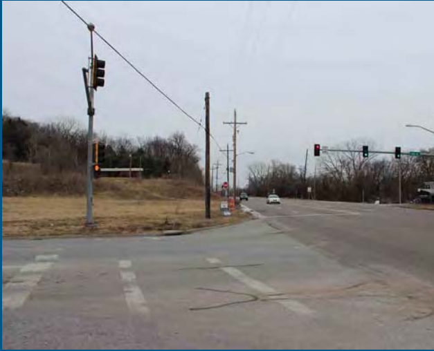
K-32 at 4th Street “Before”
